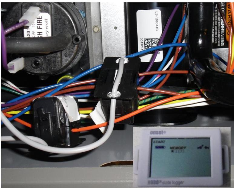
To take spot measurements of gas consumption, field staff ensured that all other gas equipment was turned off and recorded the gas consumption on the meter for a fixed period of time with the furnace on. Navigant repeated this procedure for both low and high stage for dual stage units. Field staff also installed a temperature logger near the thermostat controlling the furnace.
