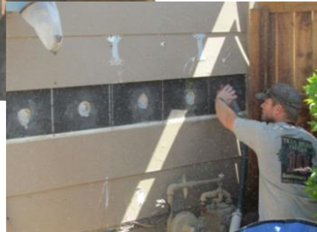
Dense packed wall insulation being installed by a technician
