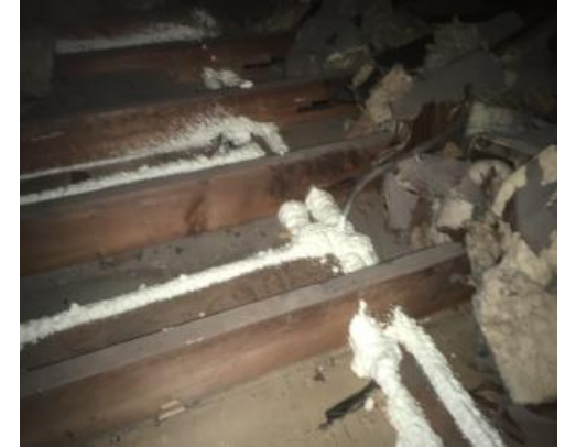
Examples of attic air sealing
