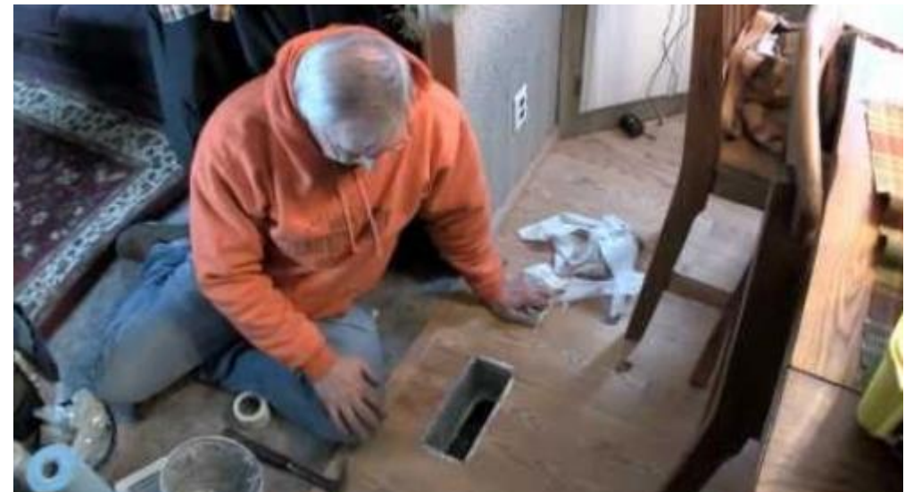
This technician is sealing duct boots in a mobile home
