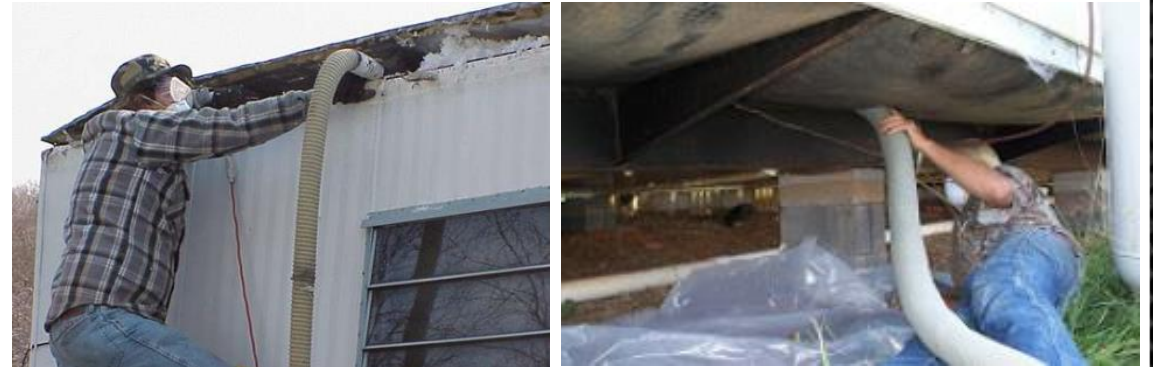
Examples of insulation techniques for mobile homes
